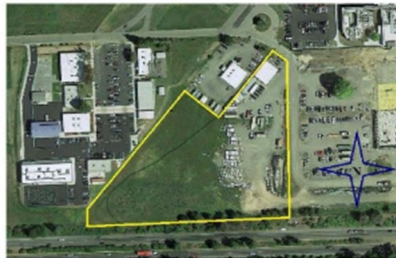
Aerial photograph with Project site outlined in yellow (April 2013 - Showing Start of Construction on Expansion Project)
